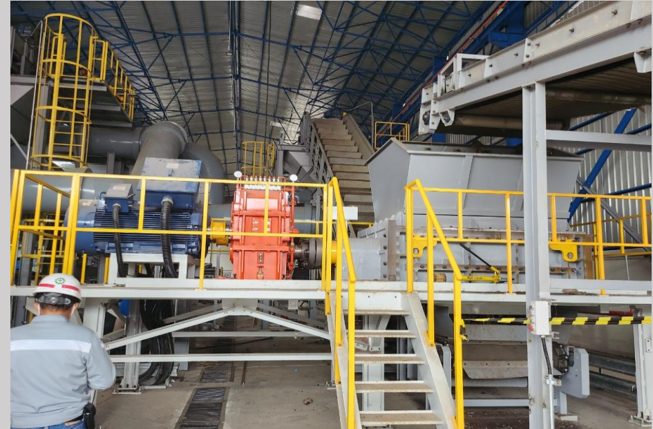
On-site Installation Status
