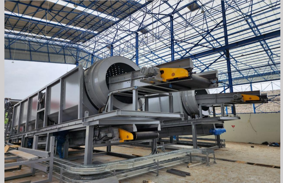
On-site Installation Status
