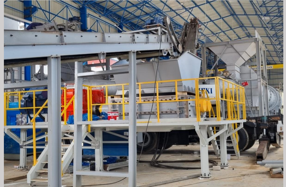
On-site Installation Status
