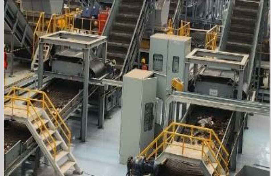
On-site Installation Status
