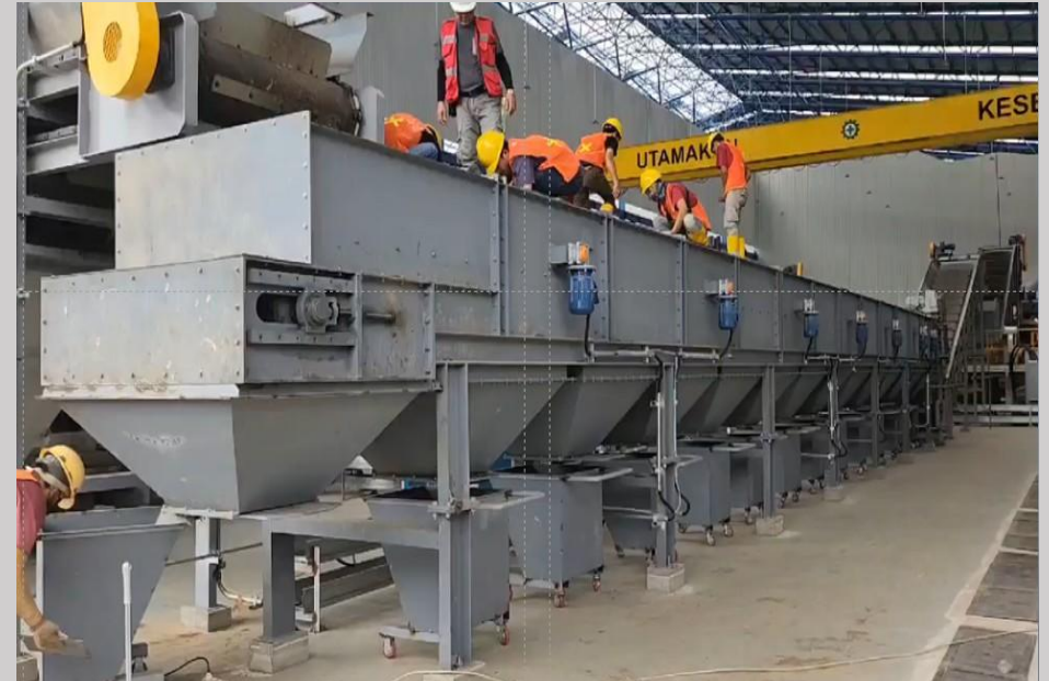
On-site Installation Status
