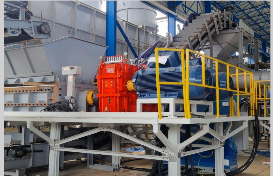
On-site Installation Status
