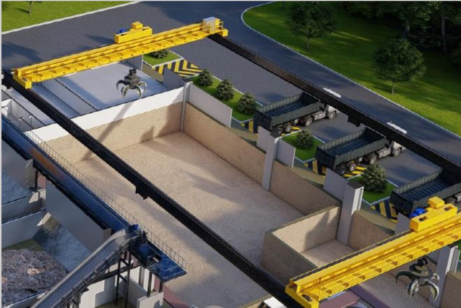
Unloading at Bunker
