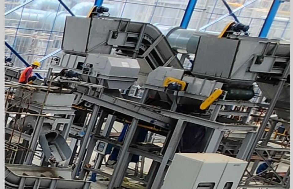
On-site Installation Status
