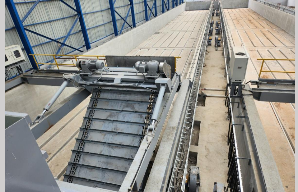
On-site Installation Status
