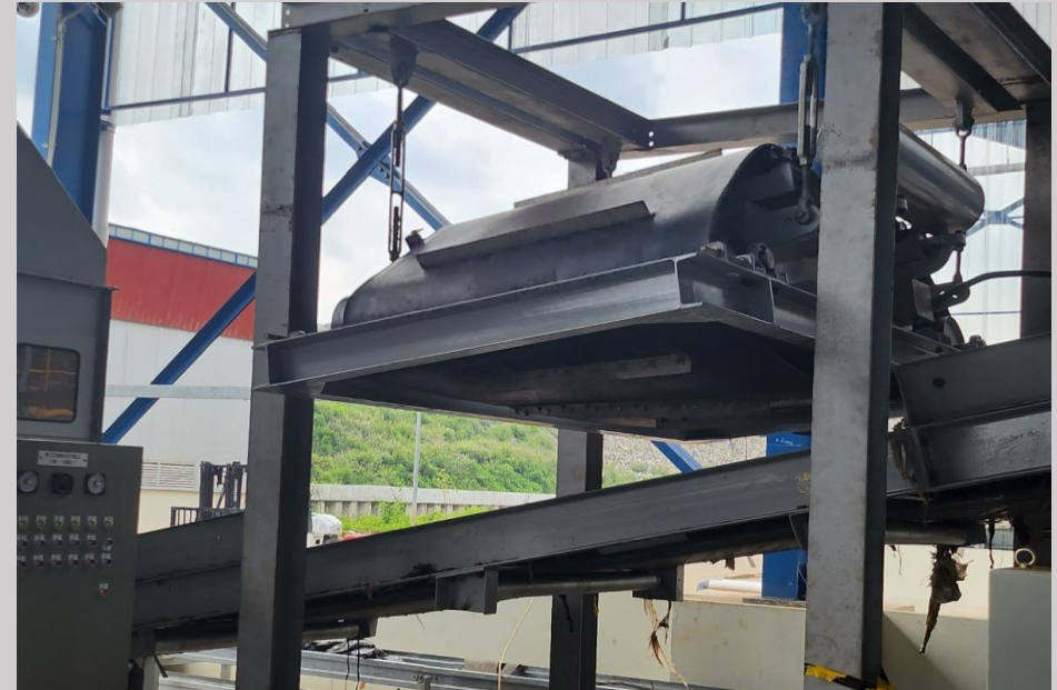
On-site Installation Status
