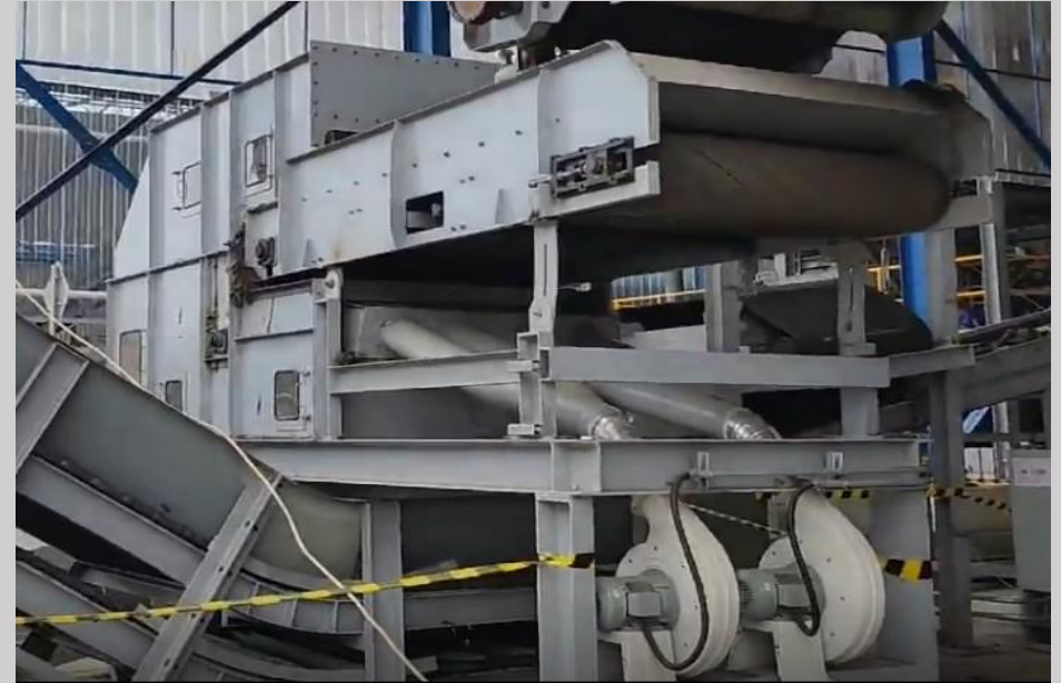
On-site Installation Status
