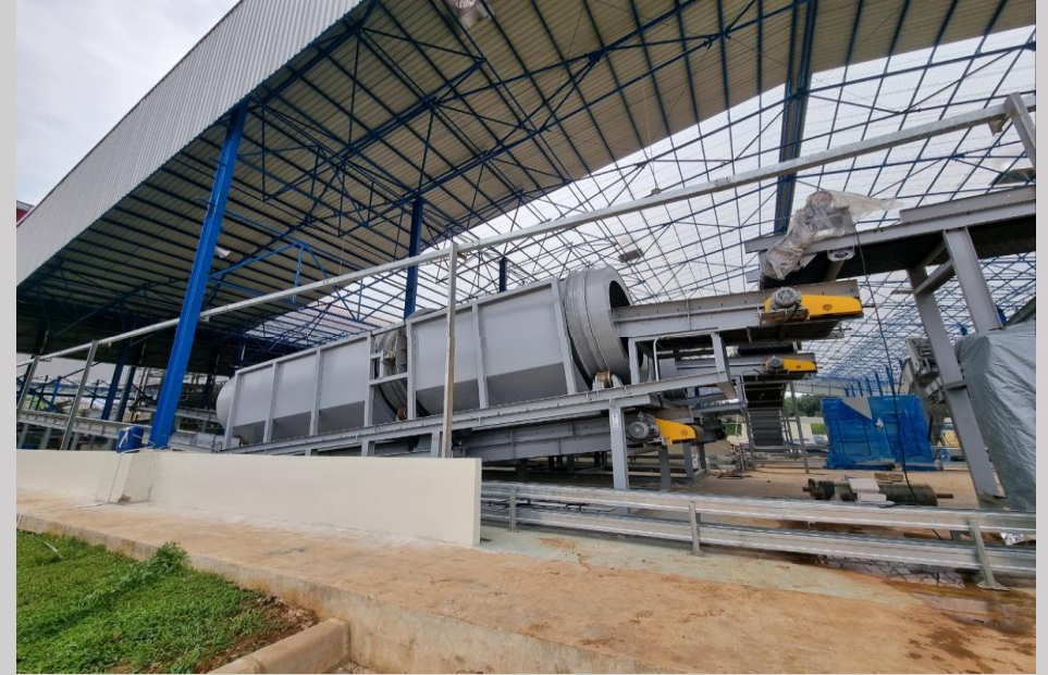
On-site Installation Status
