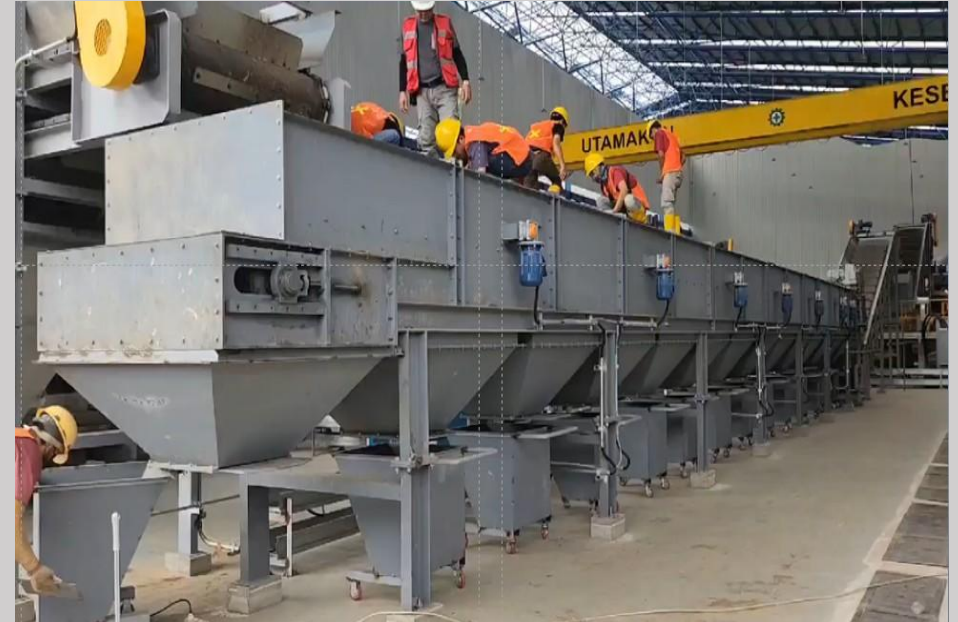
On-site Installation Status
