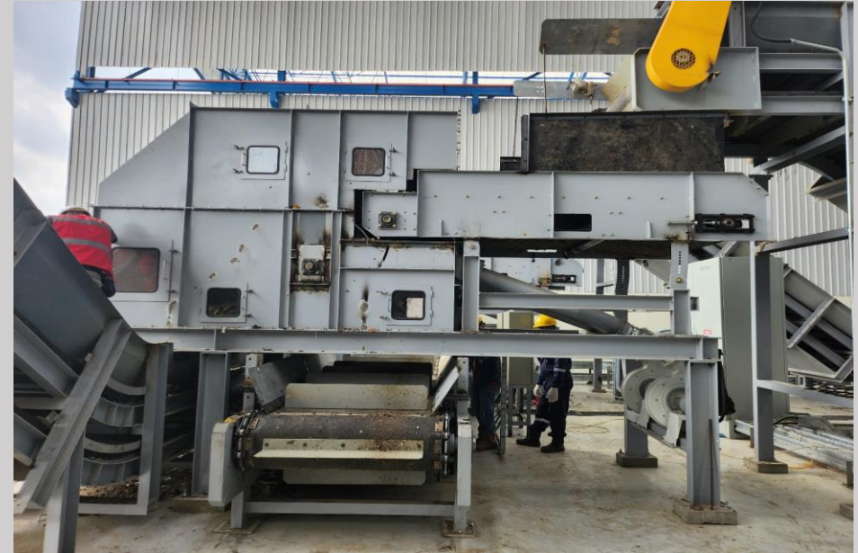
On-site Installation Status
