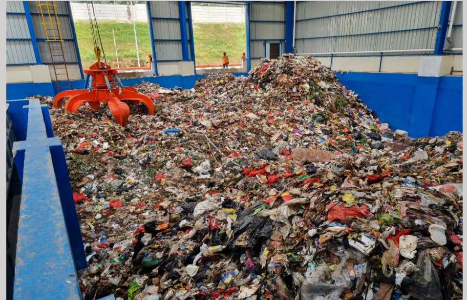
On-site Installation Status
